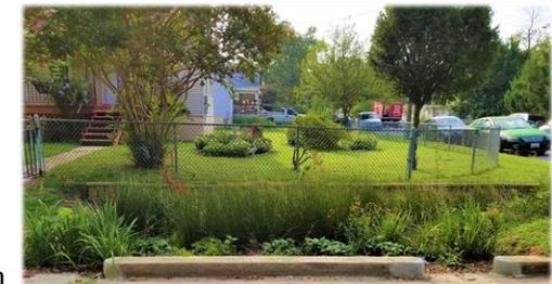
These bio-retention cells, or rain gardens, look like regular roadside green spaces, with trees and plants, but serve a very important function in the ecosystem by allowing the water to be filtered naturally through the ground. Permeable pavement in certain areas also allows water to flow into the ground. Overall, the street will capture the first 1.33 inches of rainfall during a storm, which means about 90% of all rain showers in a typical year are
